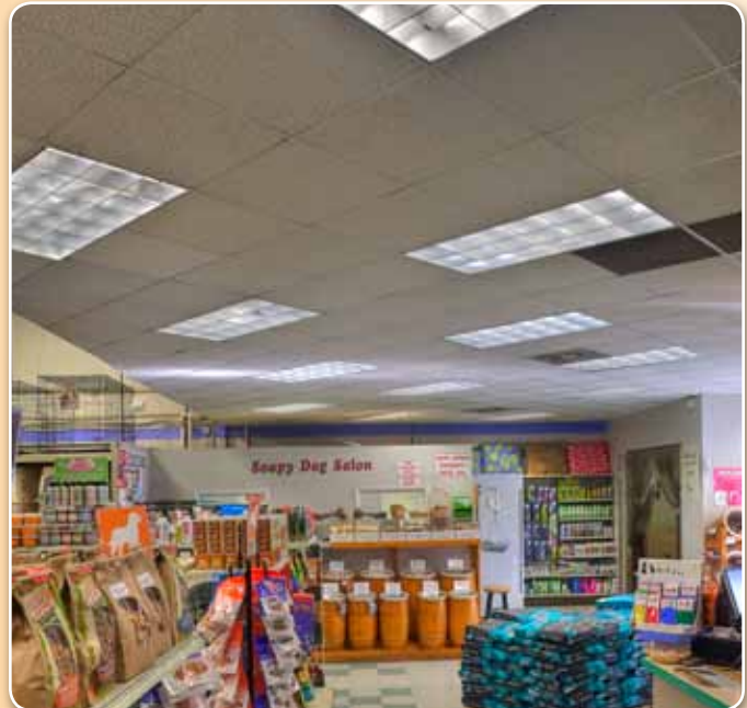
Installing new high-efficiency fixtures and ballasts has improved lighting quality.
