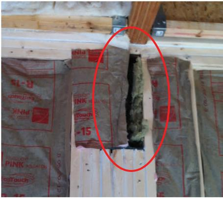
Check to ensure that steel beams connected to unconditioned space are air sealed prior to insulation. This is an ideal application for closed-cell foam.
