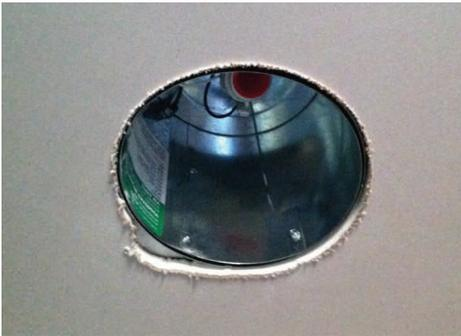
Ensure all recessed lights and exhaust fans are caulked at drywall when adjacent to unconditioned spaces.
