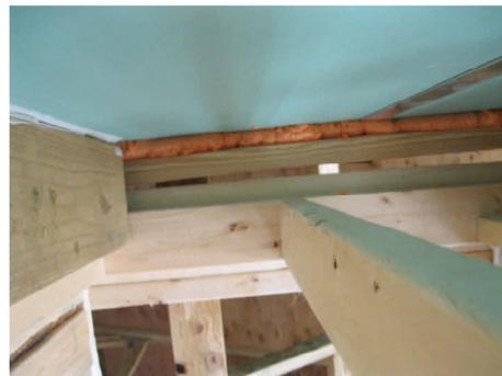
At first look, party wall appears to be properly air sealed. Looking closer reveals a larger bypass directly to unconditioned attic.
