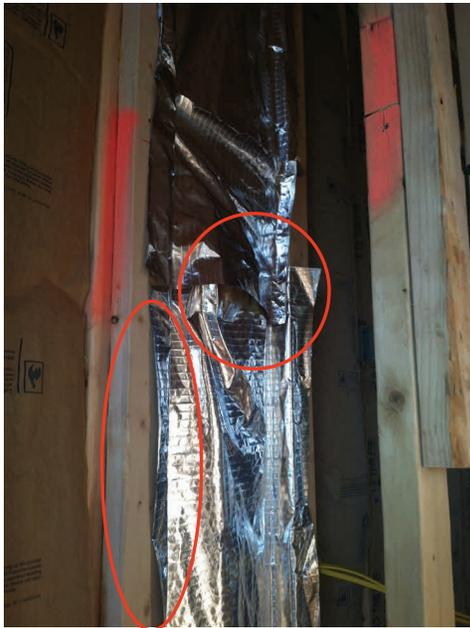
The seams and edges of this air barrier are not sealed making it ineffective.
